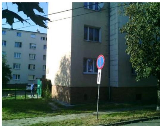
Fig. 3. Building without plinth insulation (photo: B. Ksit)
