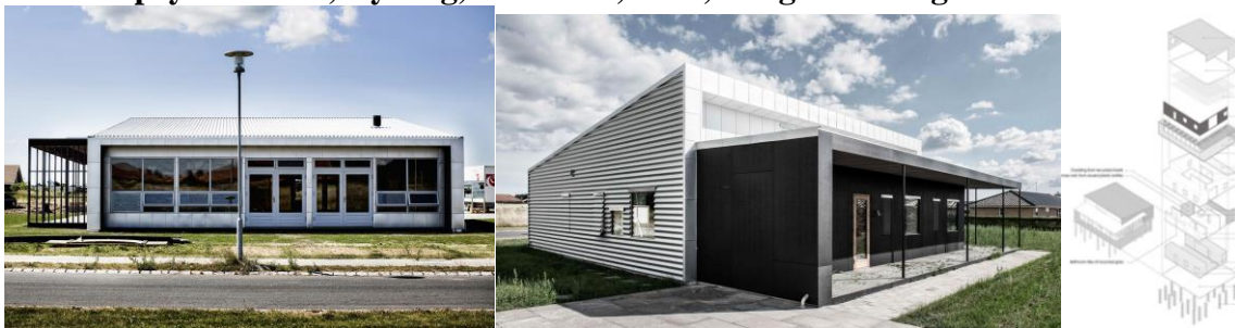
Fig. 10. Upcycle House: elevation views and structural scheme. Source: Lendager Group
