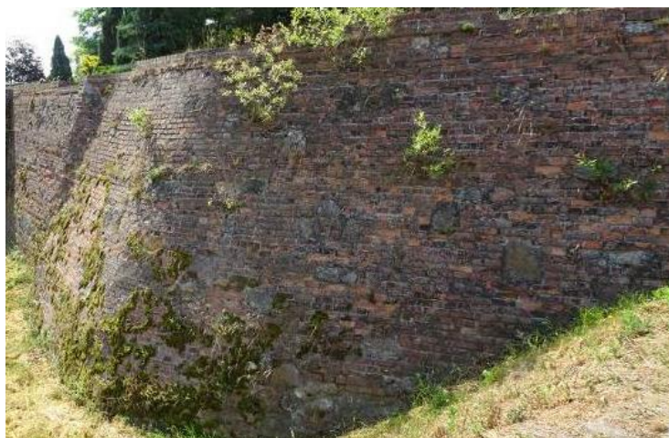
Fig. 10. Loss of masonry units and joints. Growth of planting
