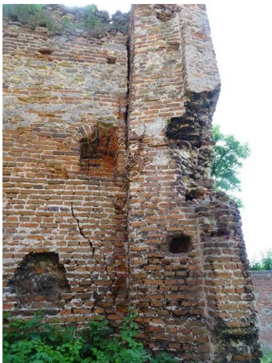
Fig. 16. Cracks and loss of masonry of the Krzepicka Gate
