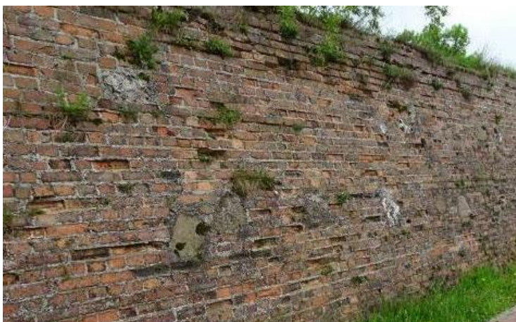
Fig. 11. Loss of masonry units and joints. Growth of planting
