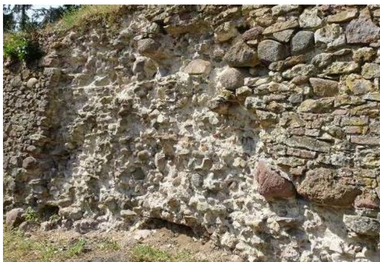
Fig. 9. Loss of masonry units and joints. Growth of planting
