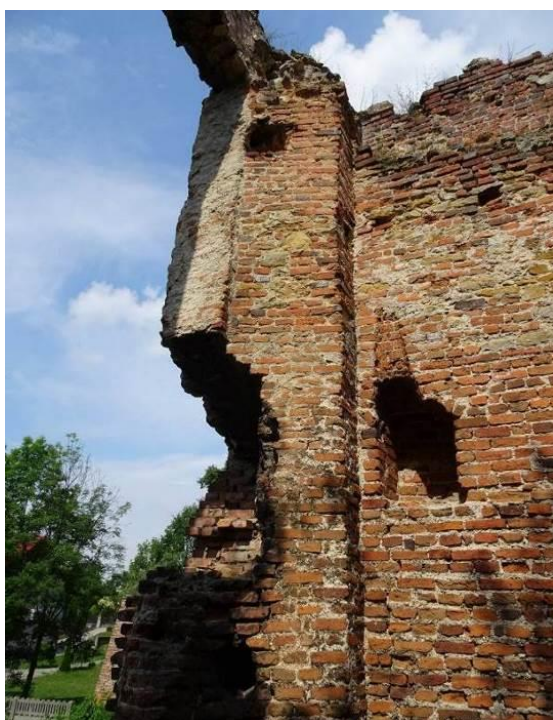
Fig. 17. Cracks and loss of masonry of the Krzepicka Gate
