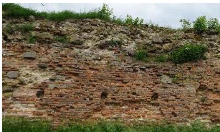
Fig. 20. Loss of masonry and joints. Cracks in masonry
