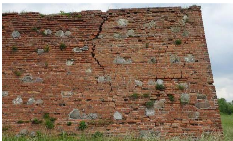
Fig. 19. Loss of masonry and joints. Cracks in masonry
