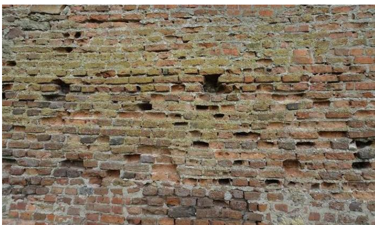
Fig. 12. Detailed loss of masonry units and joints
