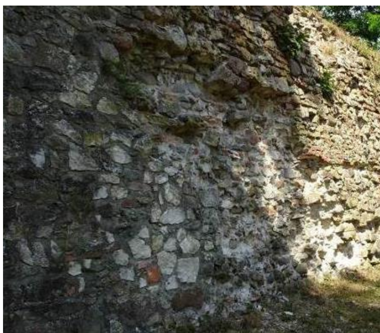
Fig. 8. Loss of masonry units and joints. Growth of planting
