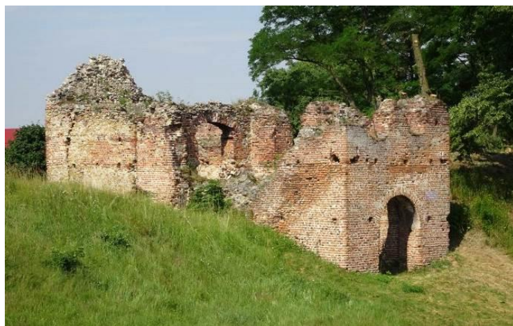
Fig. 18. Cracks and loss of masonry of the Krzepicka Gate
