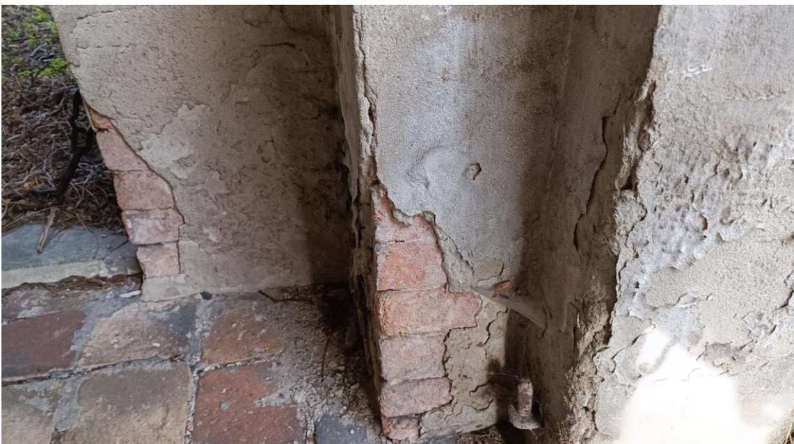
Fig. 6. Interior wall of the chapel: chipped plaster, salinity (Autor)
