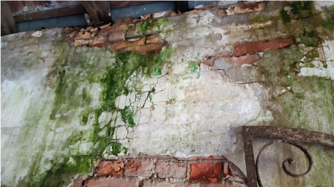
Fig. 5. View of masonry before repair: chipped plaster, salinity and biological corrosion (Autor)
