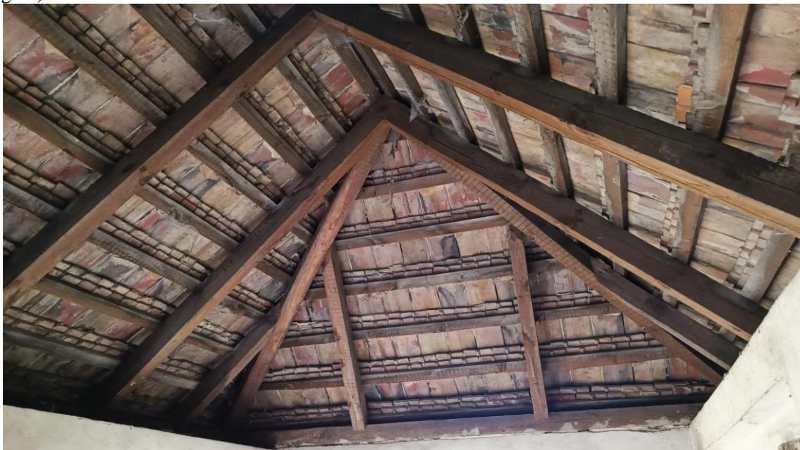
Fig. 4. Construction of the roof in the chappel (Autor)
