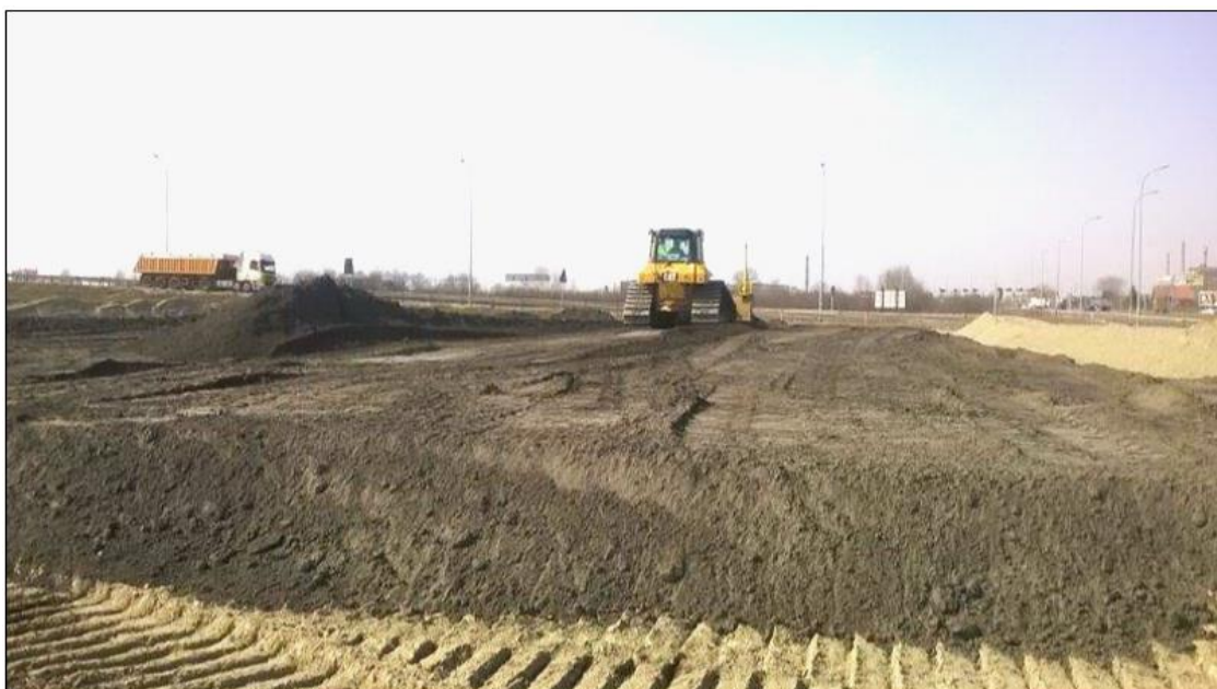
Fig. 6. Slag-ash aggregate used as road subbase. Photo by P. Calka
