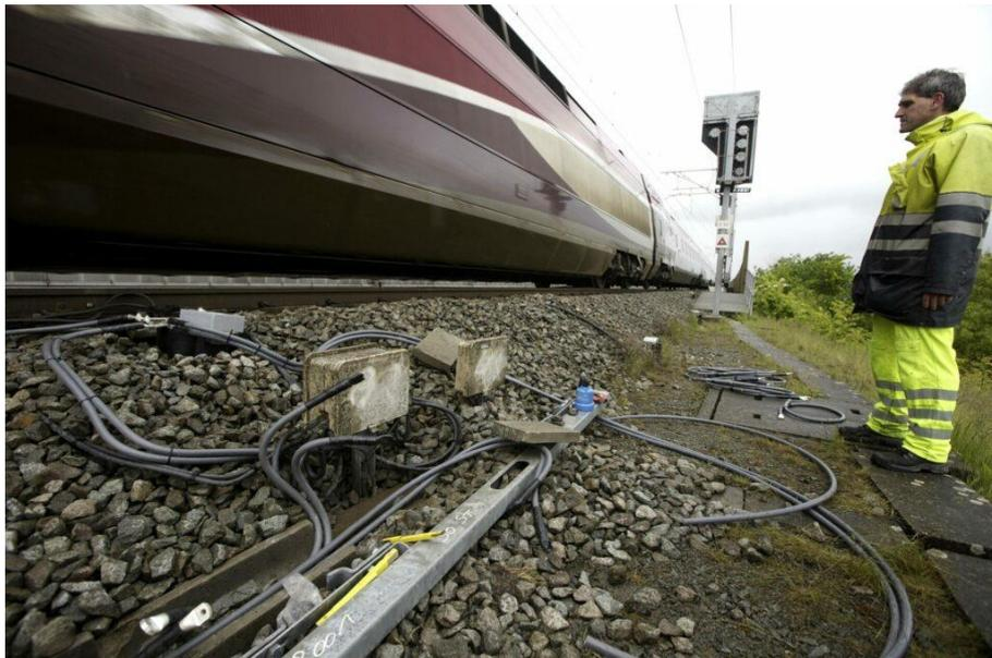
Fig. 7. Devastated cables and control command and signalling devices [36]
