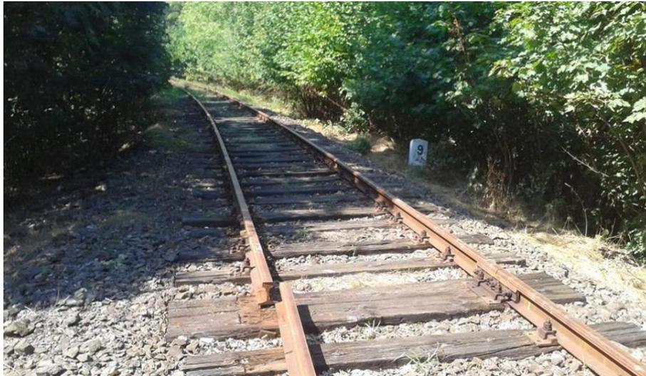
Fig. 6. The effects of theft of railroad elements (rail fastenings, screws, base plates) [39]
