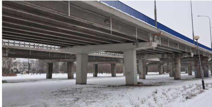
Fig. 3. Composite concrete-concrete bridge in WBS system (a flyover in Poznań).
