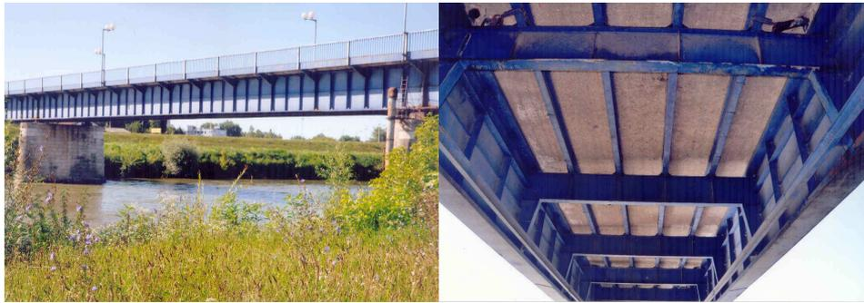
Fig. 1. Semi-composite bridge over the Sava river in Zagreb.
