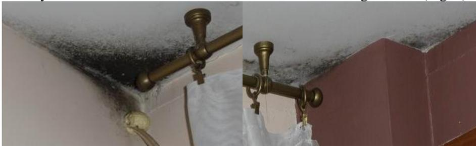
Fig. 5. Mold-covered upper wall corner below the balcony and ceiling comprising an extension of the balcony
