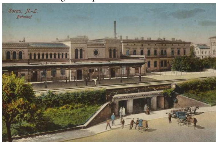
Fig. 2. Railway Station after modernization [www.zary.fotopolska.eu]
