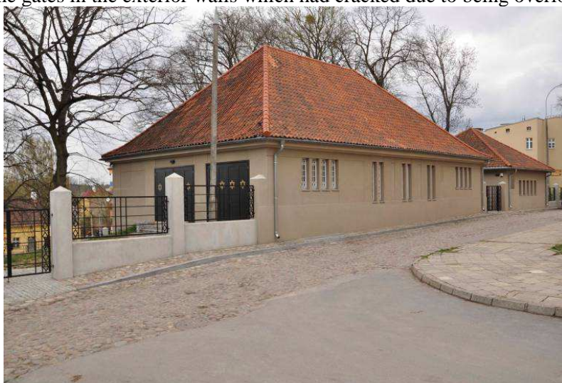
Fig. 7. Bet Tahara building complex following renovation [photograph by A. Skrzypińska, 2014]
