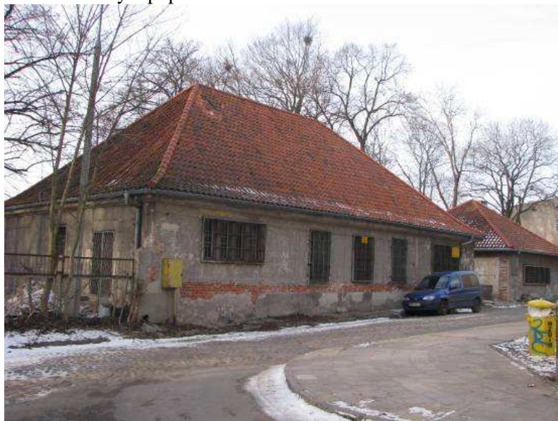
Fig. 1. View of the front elevation of the Bet Tahara prior to renovation [photograph by B.M. Deja, 2011]
