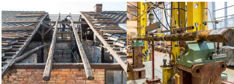
Fig. 3. Removal of rafters - barrack B-123
