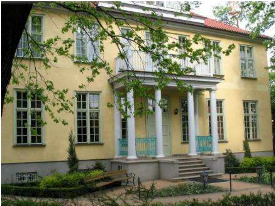
Fig. 6. Młyniska Manor after completion of construction-conservation works
