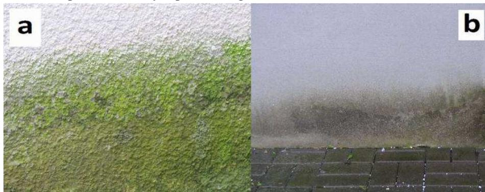
Fig. 3. Parts of the facade adjacent to the ground which the biological film for SEM observation was derived from, a - 30-year-old, non-insulated facade, very porous, b- 14-year-old facade insulated with styrofoam, covered with a thin-layer plaster
