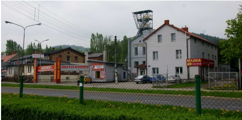
Fig. 5. The ‘Teresa’ pit bank of the closed ‘Thorez’ coal mine in Wałbrzych, with its preserved extraction tower, was sold to a private investor and turned into a car service centre (Photo: Author, 2012). However, a positive aspect of this adaptation is the small museum of technology opened on the premises.
