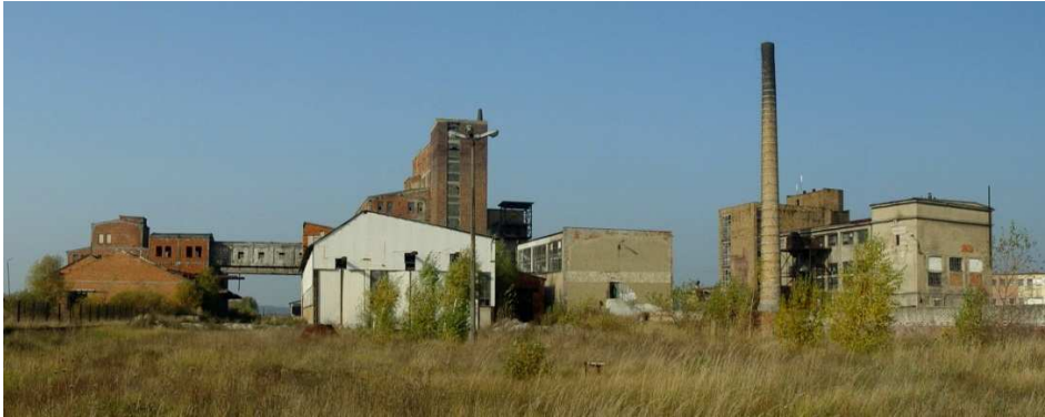
Fig. 1. The abandoned, mostly undeveloped building of the liquidated Salt Mine in Wapno. One of the deteriorating structures here houses a giant hoist, and is a protected building. (Photo: Author, 2007).
