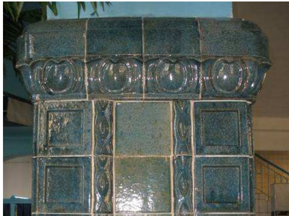
Fig. 4. Head of the pillar ceramic body of the ground floor arcade in the pool hall ( photo by the author )
