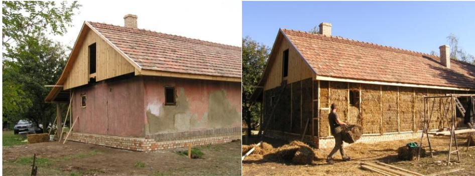
Fig. 2. Building before and during thermal renovation, Nyíregyháza, Hungary [6]
