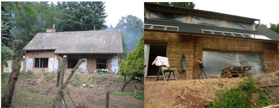
Fig. 1. The building before and during the thermal renovation with the use of straw bales, Bražec, Czech Republic (Source: [www.jakubwihan.com](http://www.jakubwihan.com))
