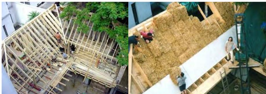
Fig. 3. The roof of the building insulated with straw bales, Vienna, Austria [10]
