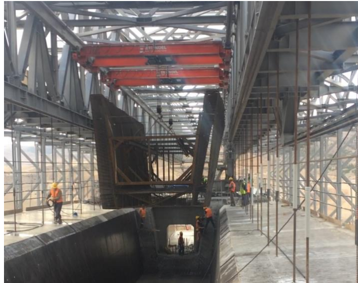
Fig. 4. M-90-S equipped with auxiliary tower cranes
