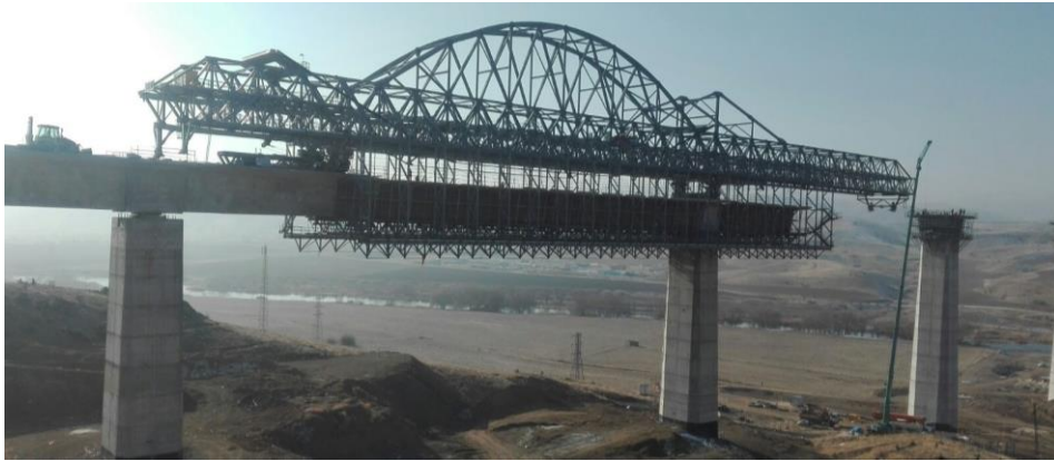
Fig. 1. Overhead MSS – M1-90-S Operating in Kirikkale, near Ankara, Turkey
