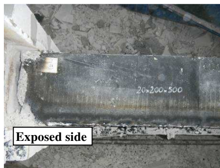
Linear joint seal No. IV extent of thermal degradation – 45 mm
