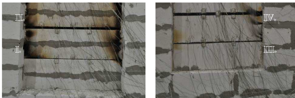
Fig. 8. Linear joint seal during the test (t = 120 min)
