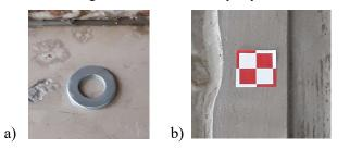
Photo 2. Network point stabilisation method controlled points, b) adjustment points
