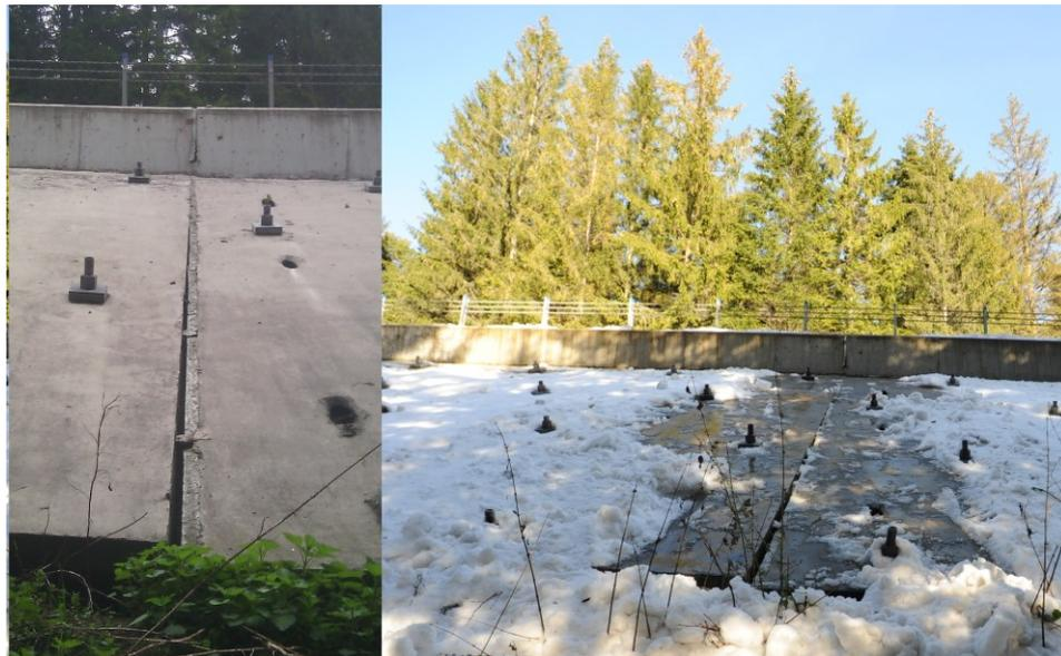
Fig. 3. Section of the failed slab of the anchored retaining structure
