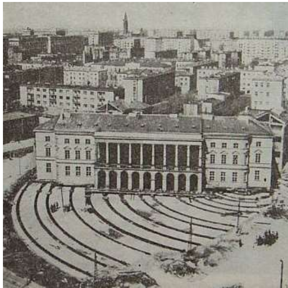
Fig. 3. Relocation of Lubomirski Palace in Warsaw in 1970 [2]
