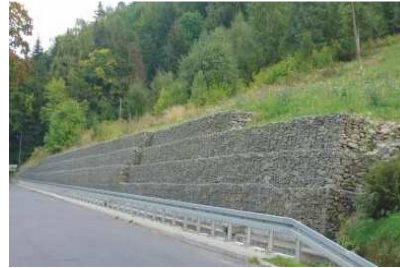
Fig.8. Retaining structure of gabion baskets [14]
