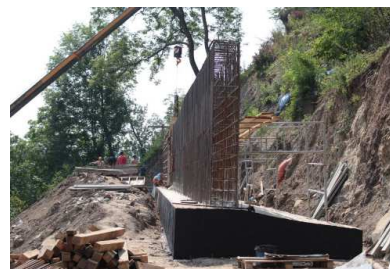
Fig. 3. Monolithic retaining being built [10]
