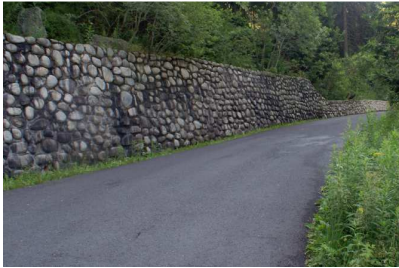
Fig. 7. Retaining structure of fieldstone [13]
