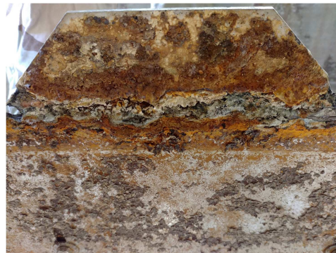
Fig. 5. Close-up onto a steel element of the drainage flume overflow ridge
