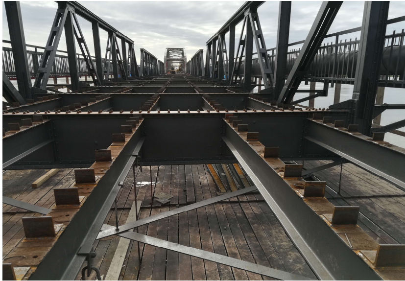
Photo 4. Replacement of the bridge slab
