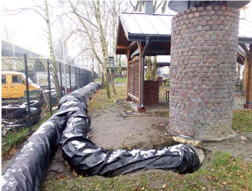
Fig. 7. The air duct installed at the surface for connecting the opening W(2015) with the opening W(2016) - the recuperation (author's photo)
