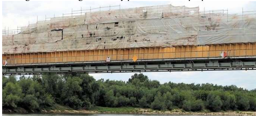
Fig. 6. View of the steel bridge during renovation - sandblasting
