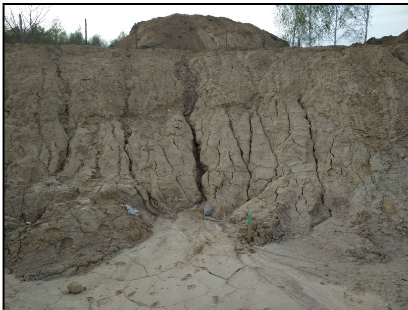
Fig. 4. Rills and gullies due to surficial runoff in silty soil [31]
