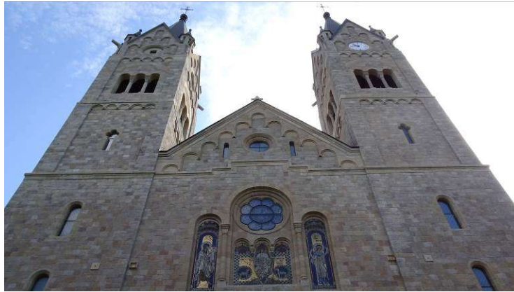
Fig. 24. The church towers before and after the renovation
