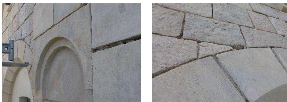
Fig. 18. Cleaned elevation and removed secondary pointing
