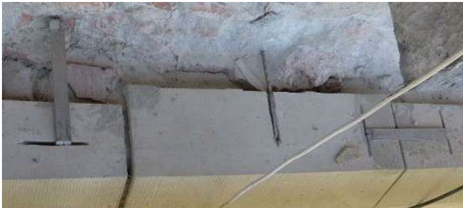
Fig. 21. Anchorage of new cornice elements in the failure zone
