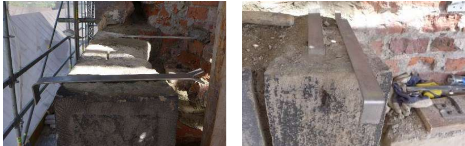
Fig. 20. Anchors for bed joints
