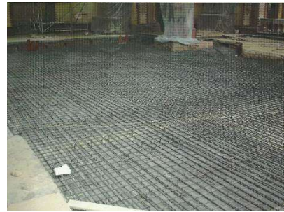
Fig. 5. Strengthening performed in the years 1986-1987: internal tie rods (left) and reinforcement of reinforced concrete slab (right)
