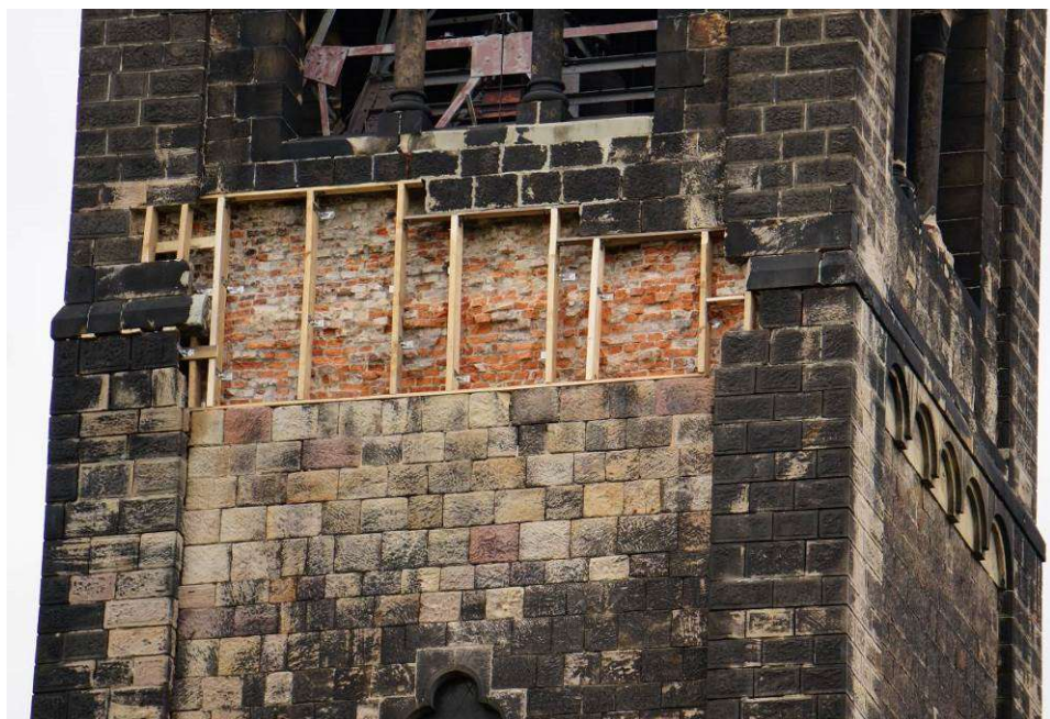
Fig. 13. Temporary protection of the debonding zone
