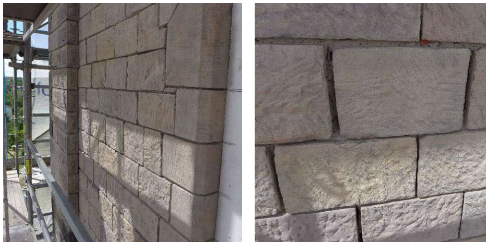
Fig. 17. Cleaned elevation and removed secondary pointing
