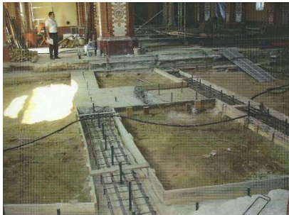
Fig. 5. Strengthening performed in the years 1986-1987: internal tie rods (left) and reinforcement of reinforced concrete slab (right)
