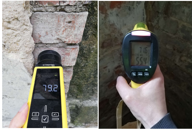
Fig. 2. Measurement of moisture content in masonry (non-invasive method)
