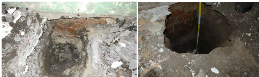
Fig. 3. Internal sample hole in the wall and basement floor
