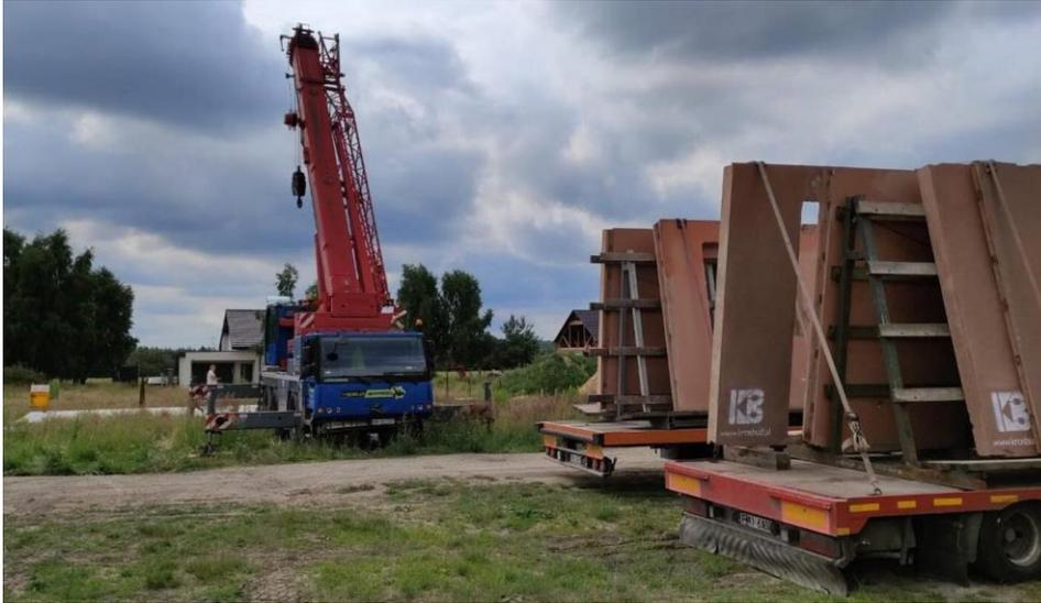
Fig. 2. Expanded clay concrete panels, authors' own photographs
