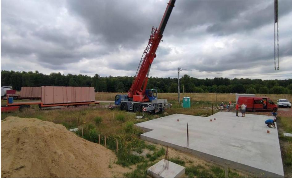
Fig. 4. Two-storey house in Pilchowiec, concrete foundation slab and installation of prefabricated walls is started, authors' own photographs
